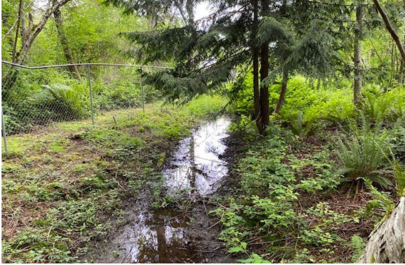
Photo 1 shows the small outlet coming out of the northwest corner of the existing detention pond.
