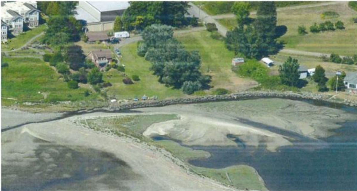
Figure 3. Oblique aerial photo excerpt of the two parcels and estuary inlet area from 2016 (WA Dept. of Ecology). House on western parcel is visible in center left and the eastern parcel extends up to the road corner.
