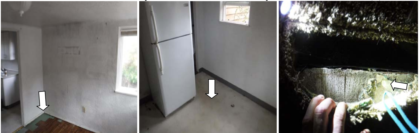
Photos 1-3: Representative Photos of Green Sheet Vinyl (Under Vinyl Plank Flooring) in Living Room (L), White Sheet Vinyl over Plywood and Concealed Green Sheet Vinyl in Kitchen (C), and White “Wood-Patterned Sheet Vinyl in SW Bedroom and Hallway on Main Floor of House (R):
