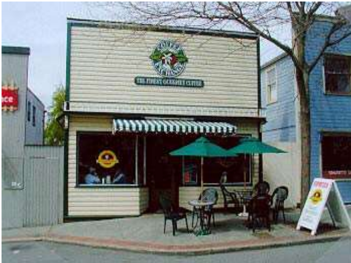
17 18 Figure IV.B.1.(a). The front of this tiny coffee shop features many pedestrian-oriented elements, 19 including weather protection, decorative lights, modest but effective ornamentation, traditional 20 siding, recessed entry, and large display windows. Note the outdoor table and chairs. Add the 21 smell of fresh brewed coffee and you have a customer magnet, not only for the coffee shop, but 22 neighboring businesses as well. 23 24
