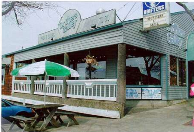
8 9 Figure IV V.B.1.(b)-1. Two examples of porches. Though simple in the extreme , the top porch 10 adds a bit of comfort and protection to an otherwise plain façade. The bottom example 11 illustrates how a covered entryway can be effectively integrated into building design. 12
