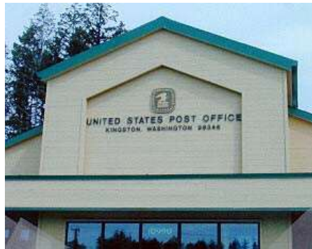
12 13 14 Figure VI.B.1.(a). The United States Post Office provides an excellent example of appropriate 15 signage. The message is clear and the lettering simple. The materials are durable and of high 16 quality. The logo is appropriate and well crafted. The sign and the building's architecture are 17 well integrated. Note how the recess in the gable provides an attractive frame around the sign 18 and adds scale and interest to the building façade in a straightforward manner.
