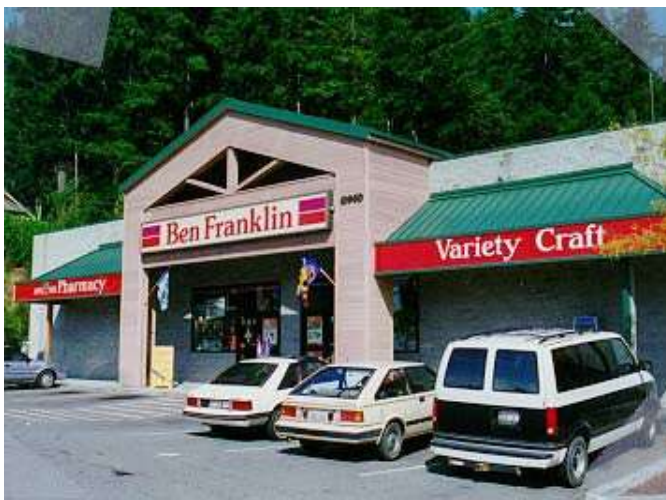
Figure IV.B.1.(d). The Ben Franklin store façade incorporates metal roof arcades and a gabled entryway to add interest and human scale to a concrete masonry unit building.
