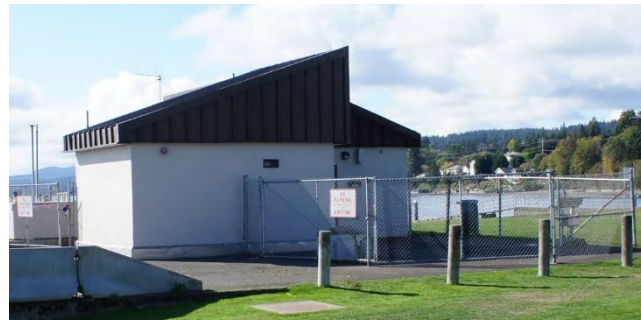
Pump Station 3 Silverdale Waterfront Park
