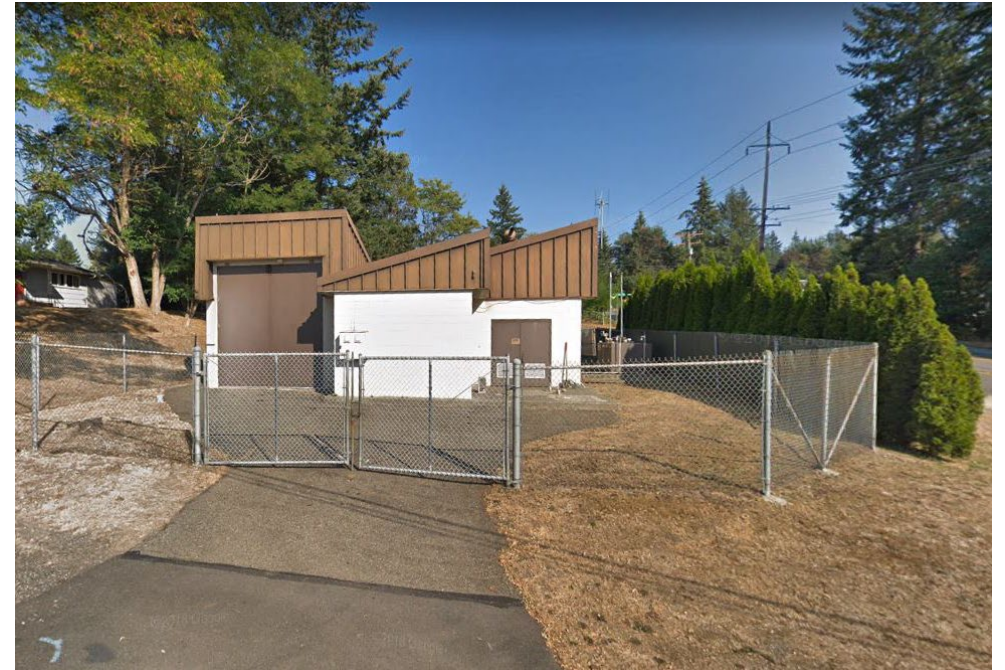
Pump Station 4 Corner of Fredrickson and Bucklin Hill Road
