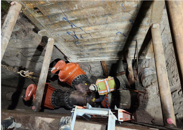
Tie-in to existing forcemain
