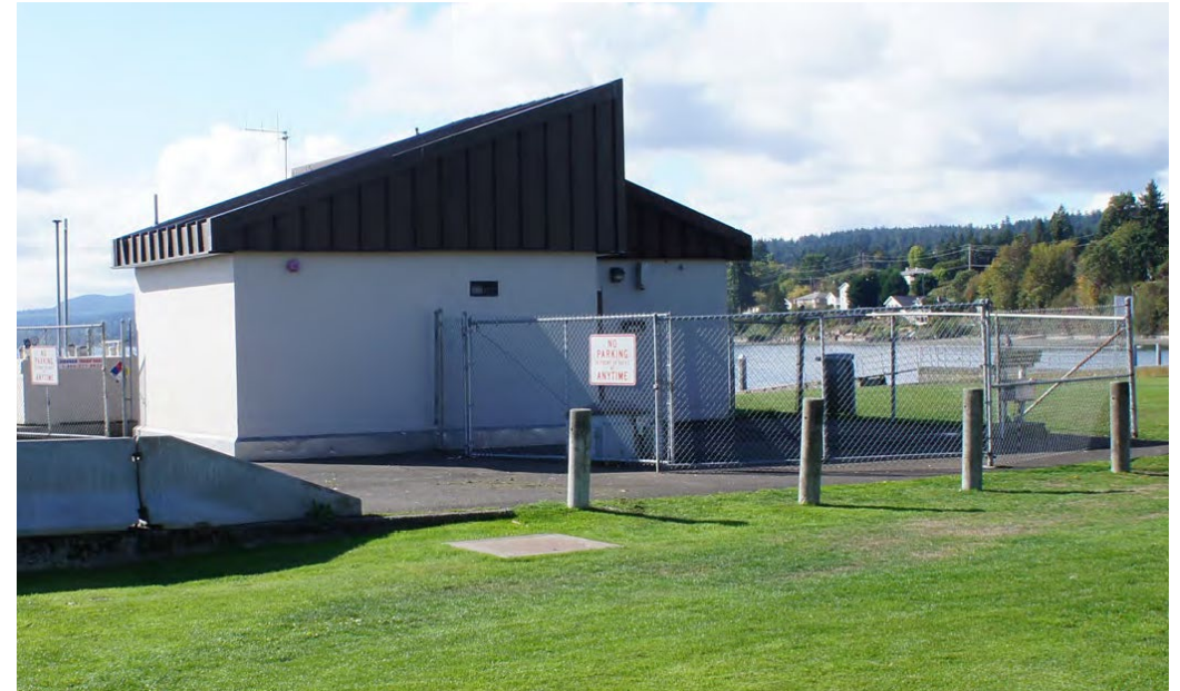
Pump Station 3 Silverdale Waterfront Park
