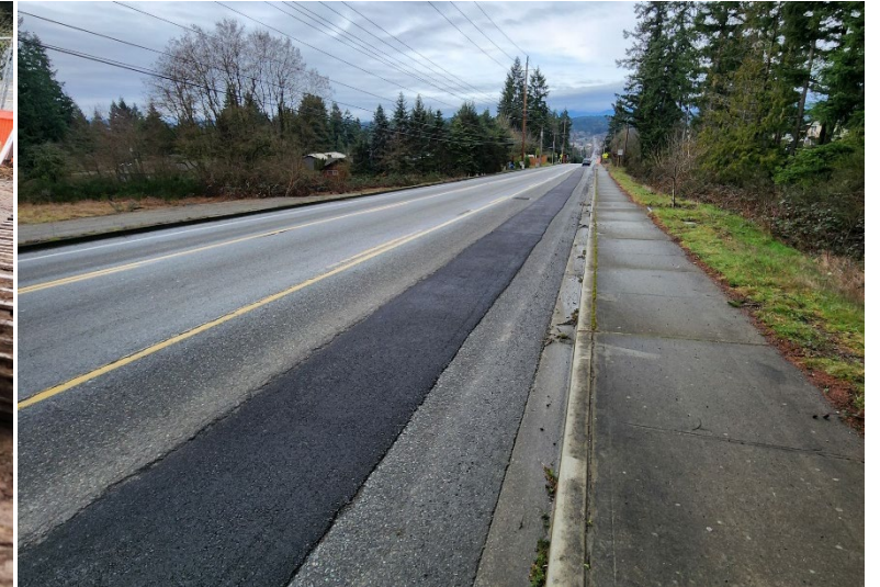
Installed forcemain on Bucklin Hill
