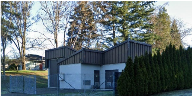
Pump Station 4 Fredrickson and Bucklin Hill Rd
