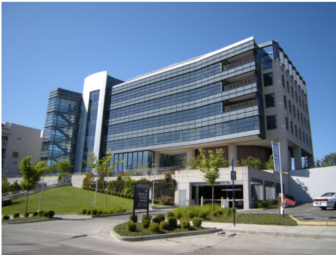
Norm Dicks Government Center in Bremerton. The county has $16.1 million in long-term obligations on this multi-agency building.
