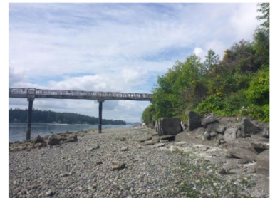
Photograph 1: New outfall structure Project area beach and shoreline bluff habitat, facing south.
