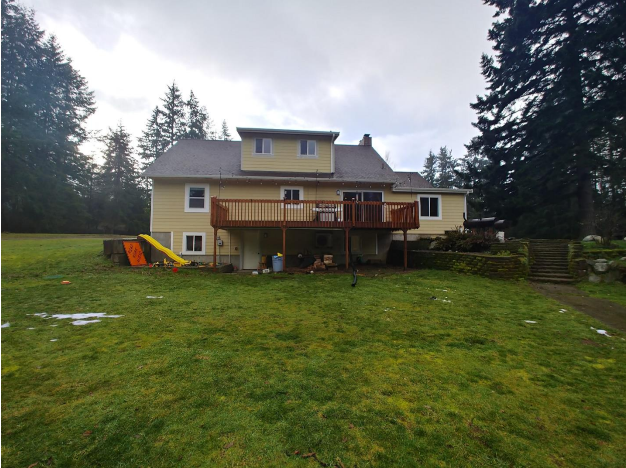
#2 Back facing NORTH
