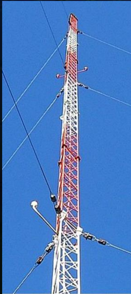
200 foot (61 m) radio mast of an AM radio station in Mount Vernon, Washington, USA, supported by three sets of 120° guy lines
