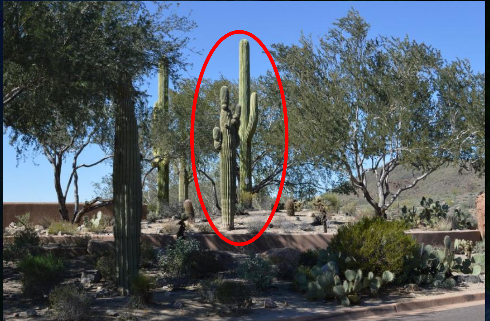
STEALTH WIRELESS SITES. SAGUARO SECOND FROM LEFT AND SAGUARO ON FAR RIGHT ARE TWO SEPARATE STEALTH WIRELESS SITES WELL DISGUISED WITH LIVE SAGUAROS. SITE IS ELEVATED FOR ADDITIONAL VERTICALITY ON A HILL OVERLOOKING A HEAVILY USED FOUR-LANE ROAD. PHOTO BY JESSE DRAKE.
