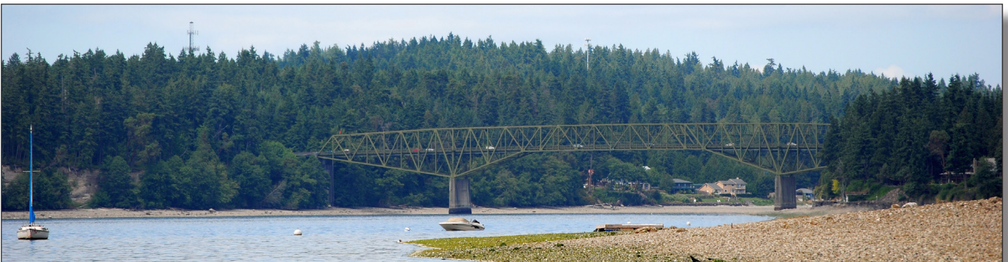
Agate Pass Bridge, Bainbridge Island
