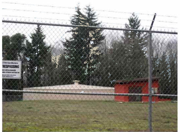
1744861 – Reservoir and Shed-GP
