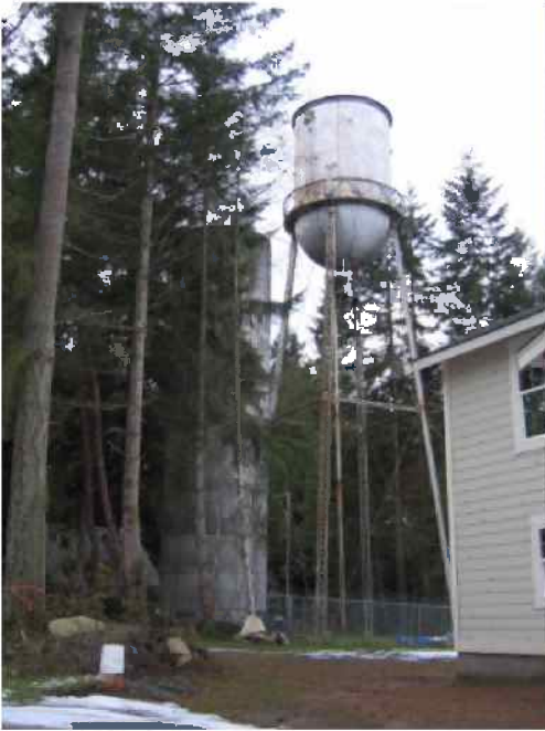
1980408 – Elevated Steel Tank
