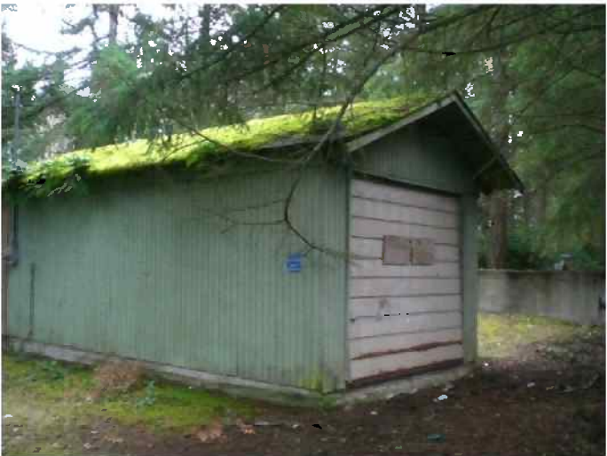
1789429 – Residential Detached Garage
