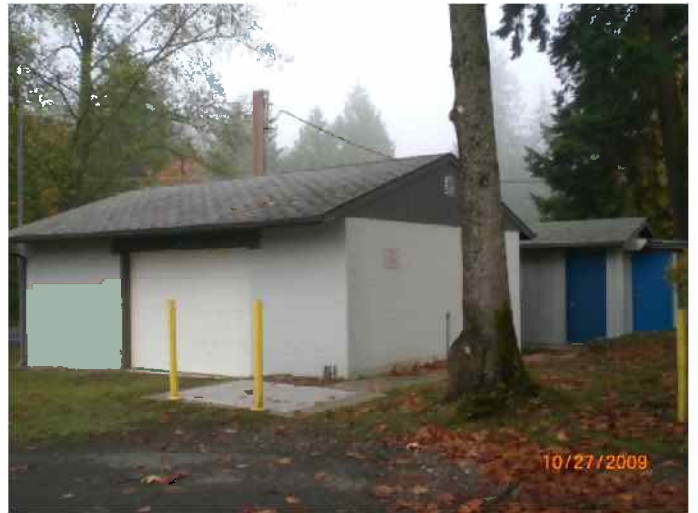
1275247 – Residential Detached Garage
