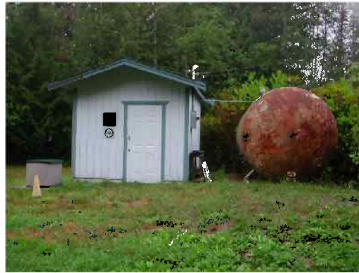
1230374 – Shed –GP Tank is???
