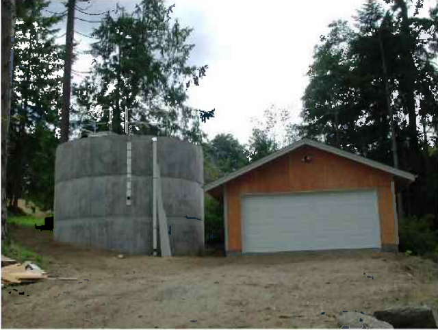
2299253 – Concrete tank with Residential Detached Garage
