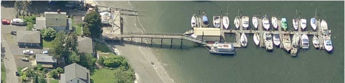
Figure 5.2.1 Keyport Marine Services facilities.
