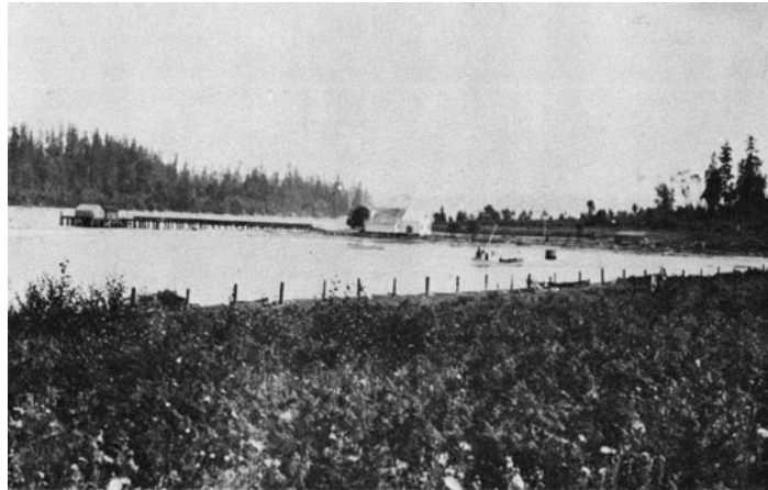
Figure 5.1.3 Original Keyport Store & Community Dock.
