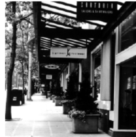
Transparent canopies provide protection from the rain but allow light to filter through.
