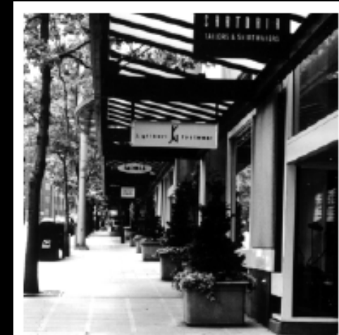
Transparent canopies provide protection from the rain but allow light to filter through.
