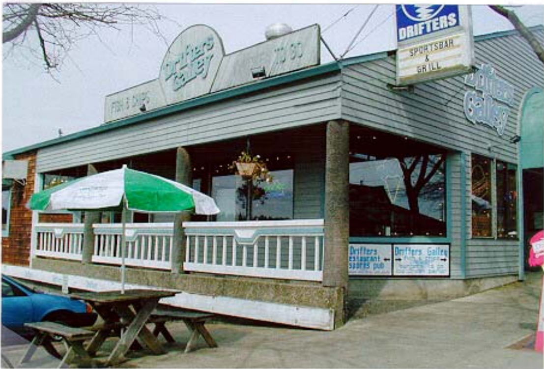
Figure V.B.1. (b). Two examples of porches. Though simple in the extreme, the top porch adds a bit of comfort and weather protection to an otherwise plain façade. The bottom example illustrates how a covered entryway can be effectively integrated into building design.
