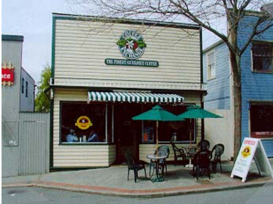
Figure IV.B.1.(a). The front of this tiny coffee shop features many pedestrian-oriented elements, including weather protection, decorative lights, modest but effective ornamentation, traditional siding, recessed entry, and large display windows. Note the outdoor table and chairs. Add the smell of fresh brewed coffee and you have a customer magnet, not only for the coffee shop, but neighboring businesses as well.
