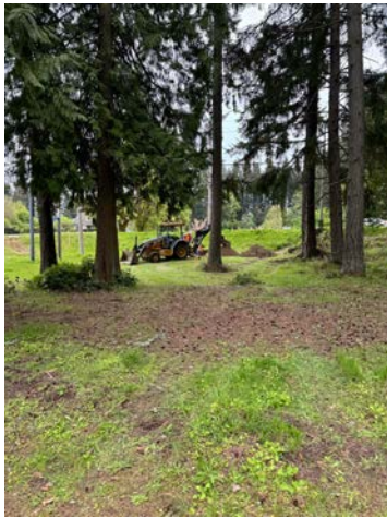
Gas line installation
