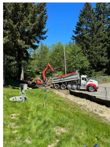
Site work began
