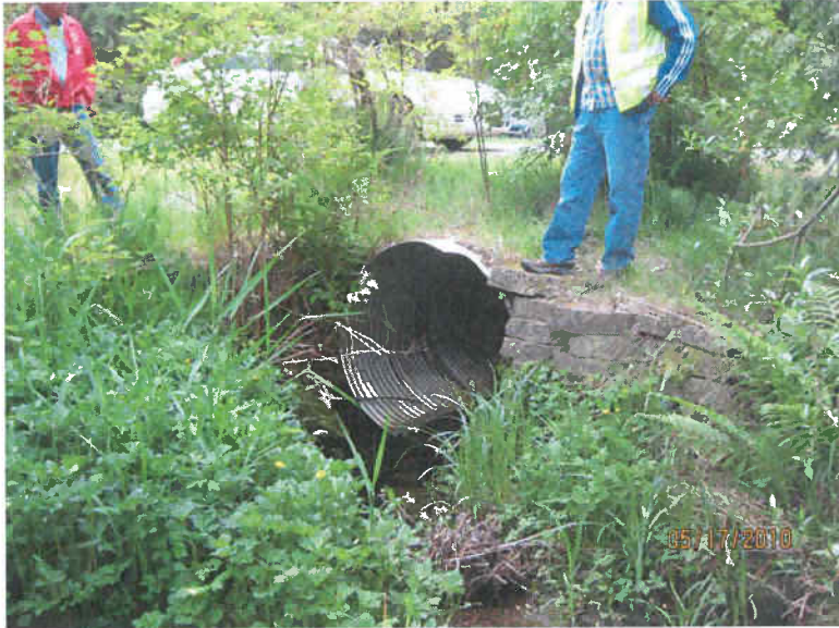
Existing Culvert at Shadow Glen Road (Upstream)
