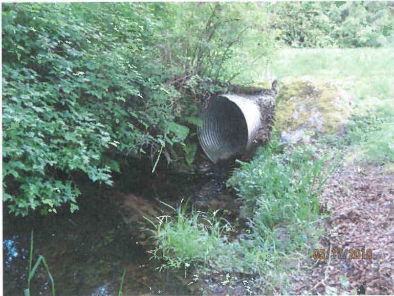
Existing Culvert at Shadow Glen Road (Downstream)
