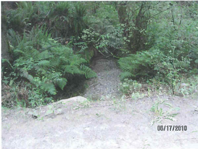
Existing Culvert at Sunde Road (Upstream)
