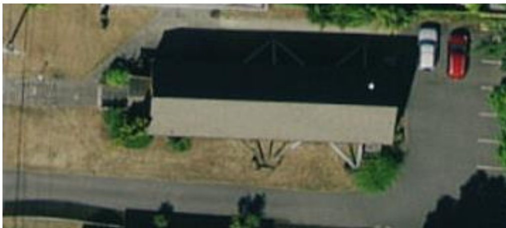
Log Church/Storage: 717 Sidney Ave Port Orchard, WA 98366
