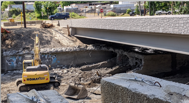
Culvert removal on Chico Way
