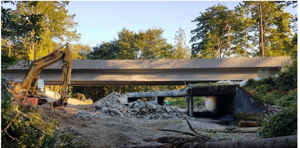
Before any work in the stream, the water was bypassed around the site using a pump. Fish were removed and relocated to safe waters.
