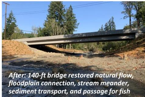
*After: 140-ft bridge restored natural flow, floodplain connection, stream meander, sediment transport, and passage for fish*
