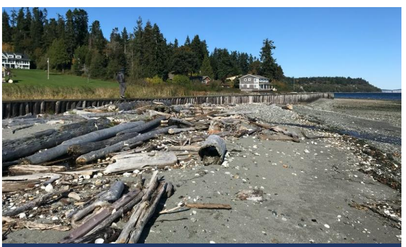
Rose Point Embayment Restoration – remove a creosote bulkhead and reconnect a stream.
