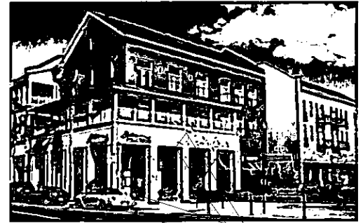
EXAMPLE OF PROMINENT CORNER ARCHITECTURE
