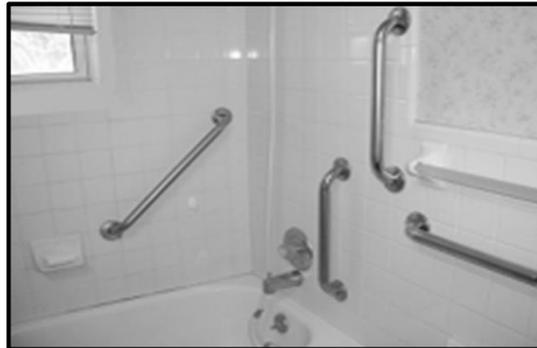
Grab bars on the shower/tub wall can help a person safely lower themselves onto a seat or into the water, and make getting out much safer.
