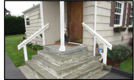
The absence of handrails on a stairway can be a real danger to the elderly or infirm. The most common point of entry to your home is from the garage, yet very few homes have any handrails on these steps. Often the steps off a porch or deck have no railing.
