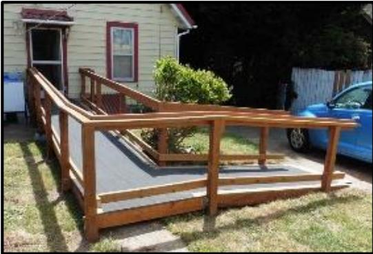
Ramps are custom built using pressure treated (weather resistant) lumber. They can be straight, L-shaped, or switchback to fit the site.
