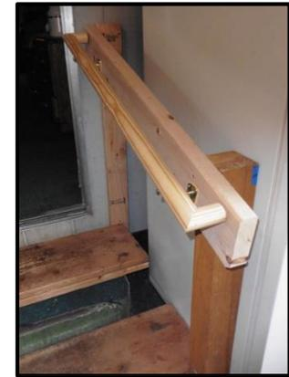
This simple, low cost handrail provides a sturdy gripping surface.
