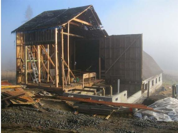
Additional work includes removal of barn debris, expanded structural damage interface with 1946 barn, and electrical panel relocation and upgrade.
