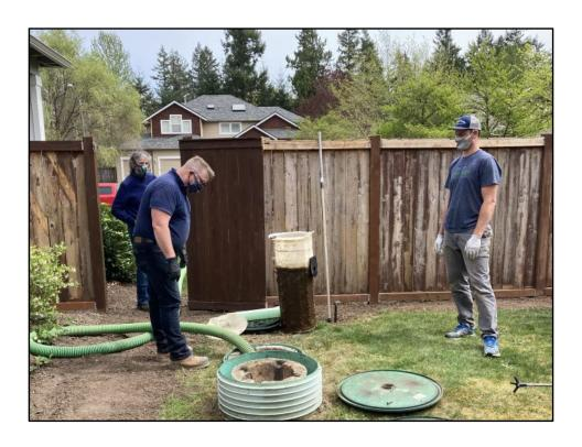
Even with regular operation and maintenance, alternative systems can still get thick scum and sludge. One of our colleagues had high scum and sludge in one compartment. The pumper didn't empty it during two prior visits because they didn't want to remove internal parts. During the next checkup, it was still 80-90% full of solids – yikes – that's not good! If you have an alternative system like this, check with the pumper to see if your maintenance person needs to be on hand during pumping.
