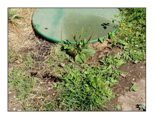
See the stained area on the green septic tank riser and signs of moisture on the otherwise dry ground. These are signs of a septic tank overflow that has partially dried.
