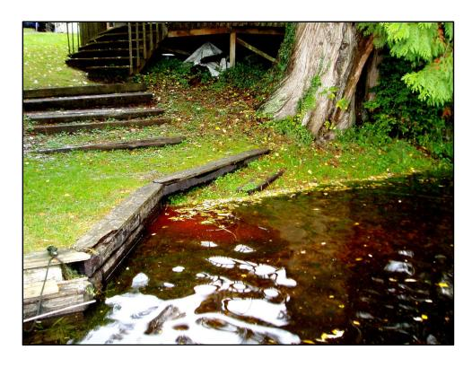
Here we confirmed that sewage was leaking into the lake by flushing red dye in the house toilet and seeing it come out in the lake.
