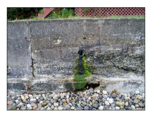
We found high bacteria counts at this bulkhead drain and dye testing the house confirmed it was sewage leaking out on the beach.
