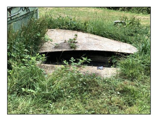
This tank is a hazard because it is open to the ground surface where people and pets can fall in, and flies can transport waste out.
