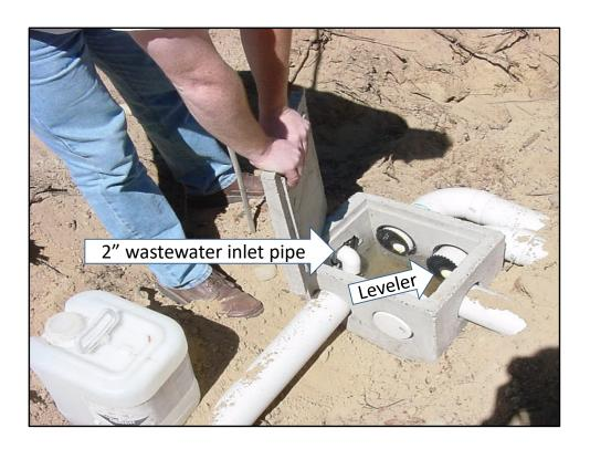
The wastewater then leaves the tank, flowing through a watertight pipe into a distribution box. You can see that 2-inch pipe here.
