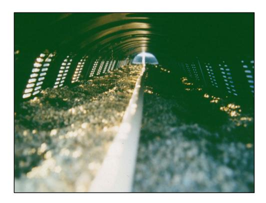
This is a rare look inside a gravelless drainfield. These chambers are used when clean gravel is hard to find or on sites where access is difficult.
