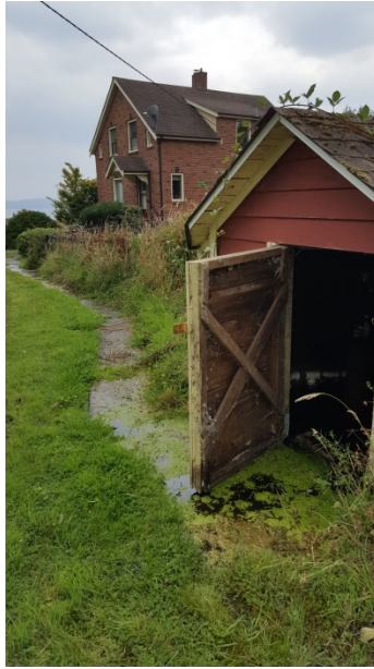
Figures 2 and 3. View inside well housing structure, showing leaking well-head (left). View looking south showing water flowing downhill from leaking well-head (right).
