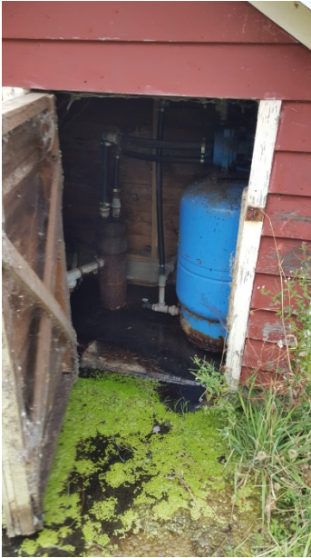
Figures 2 and 3. View inside well housing structure, showing leaking well-head (left). View looking south showing water flowing downhill from leaking well-head (right).
