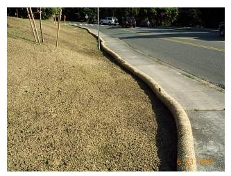
Example of shallow gradient slope with berm installed at downgradient edge to minimize siltladen runoff onto the sidewalk.
