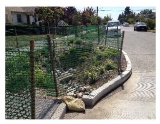
Sand bags prevent silt-laden flow from entering the bioretention BMP. Green construction fencing prevents compaction due to foot traffic. Volume II Figures
